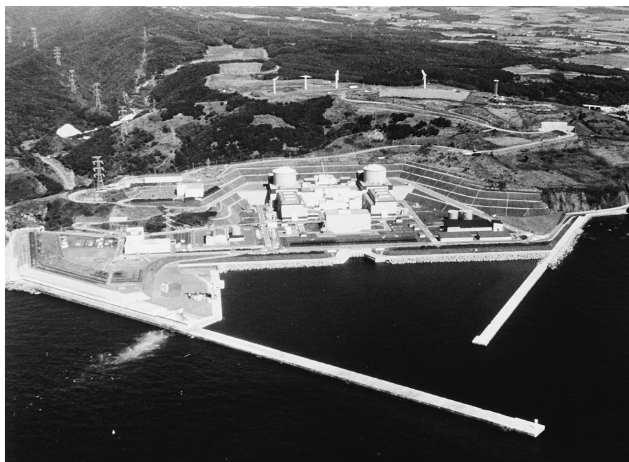
Tomari NPS of Hokkaido Electric
